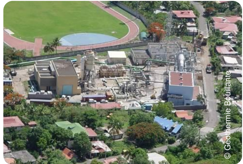
Bouillante geothermal power plant, Guadeloupe
